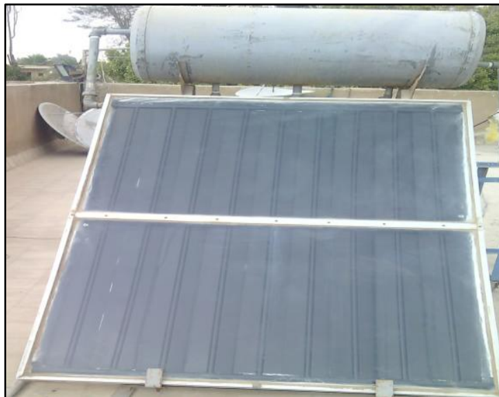
Fig.4.5: Flat plate collector
