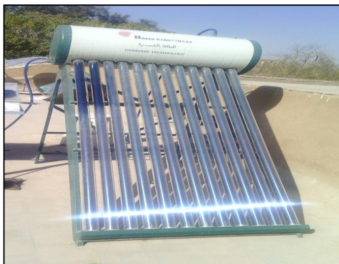
Fig.4.4: Evacuated tube collector
